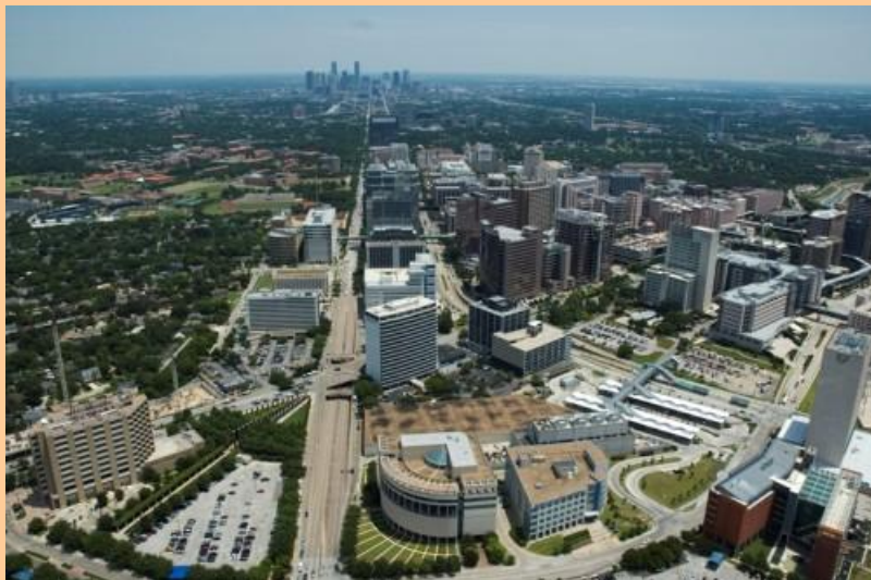
The Thermal Energy Corporation's new CHP plant will provide reliable, efficient energy to the Texas Medical Center.
